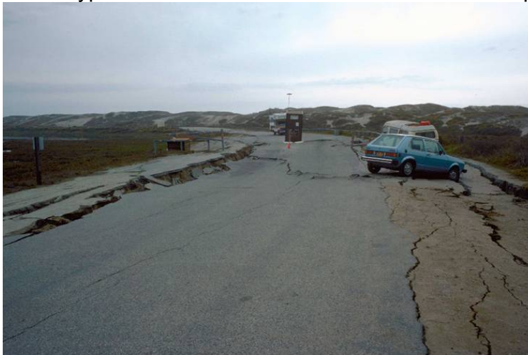
Picture 18: Lateral spreading at Moss Landing (Monterey Bay) due to the 1989 Loma Prieta Earthquake
