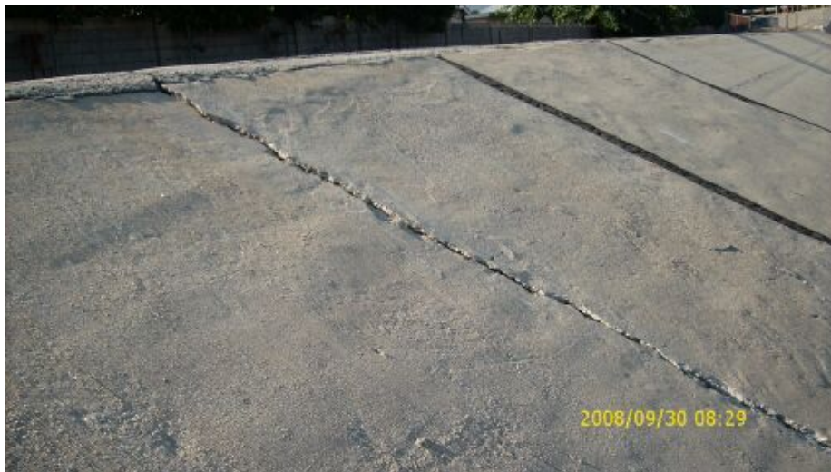
Picture 5: Vertical cracking along Coyote Creek repaired by FMD routine maintenance
