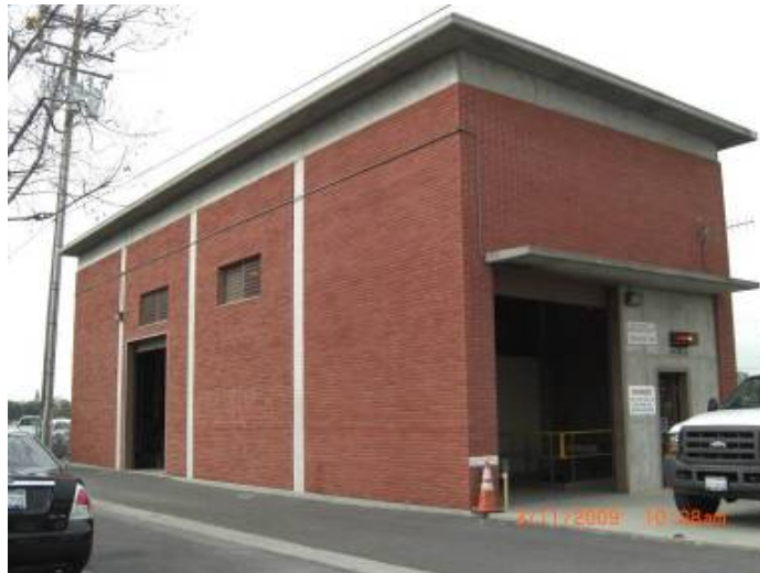
Picture 14: Los Altos Pumping Plant along Cerritos Channel in Long Beach
