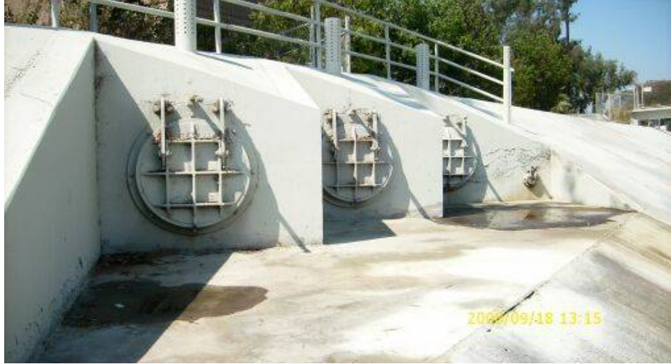
Picture 13: Flap Gates associated with the Claretta Pump Plant along Coyote Creek
