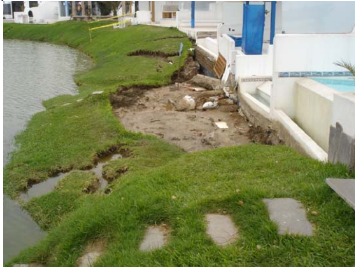
Picture 20: Lateral spreading in Las Lagunas, Peru following the August 2007 8.0 Magnitude earthquake in Pisco, Peru
