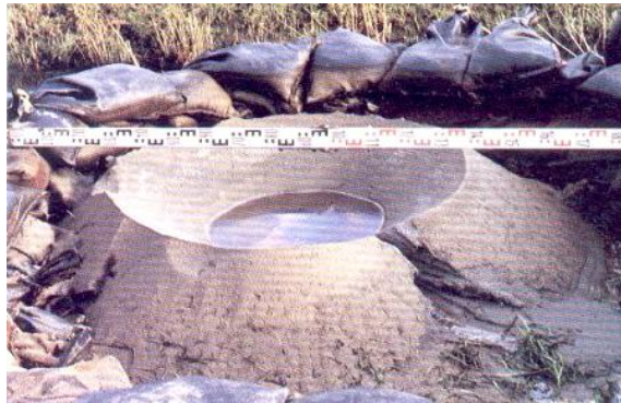
Picture 17: Sand boil downstream of river dyke in Mai-Dong Vietnam, 1997
