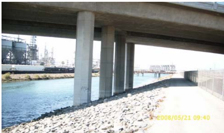
Picture 9: Anaheim Street Bridge piers installed within the Dominguez channel levee slope
