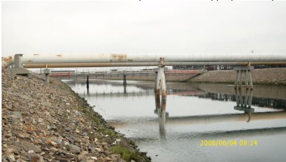
Picture 8: Dominguez Channel, free of slope vegetation
