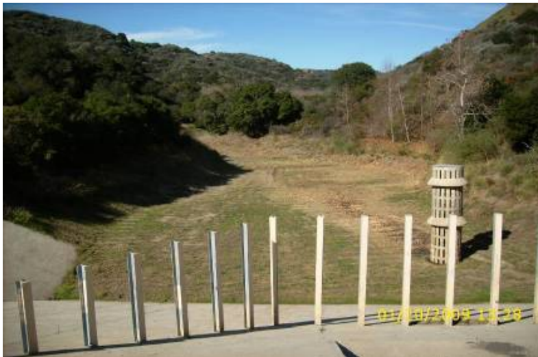
Picture 15: Sullivan Debris Basin in Rustic Canyon
