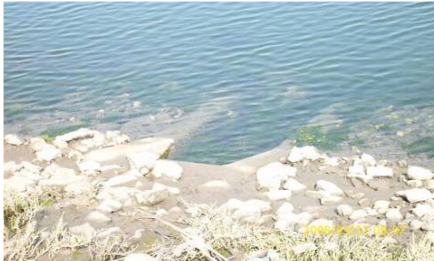
Picture 11: Submerged subdrain along Dominguez Channel
