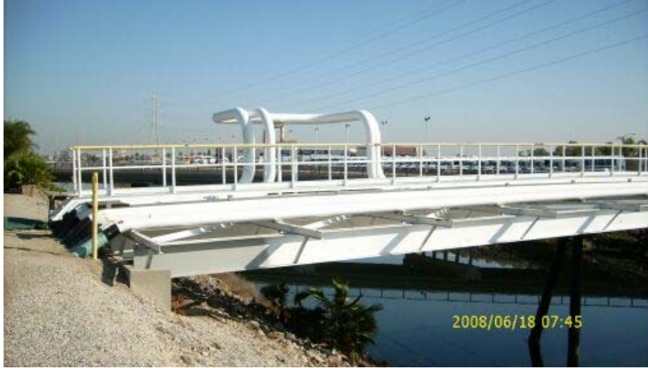
Picture 10: Utility bridge installed at the top of the Dominguez Channel levee slope
