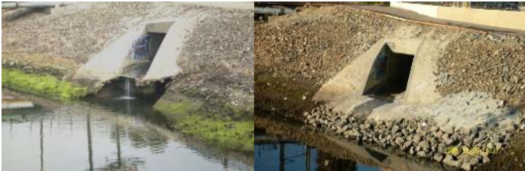
Picture 6: Erosion repair of Project 1202 outlet along Dominguez Channel
